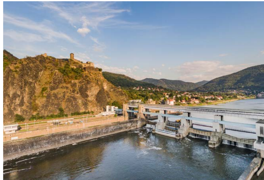
7 Střekov Castle & Locks nice walking excursion around the river / 40 mins from the city centre
